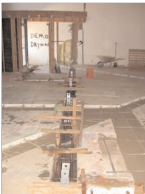
The new dojo, under construction
